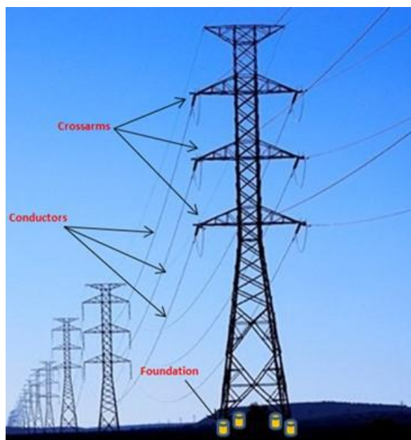
Figure 9: Typical Structural Components of DCT towers
